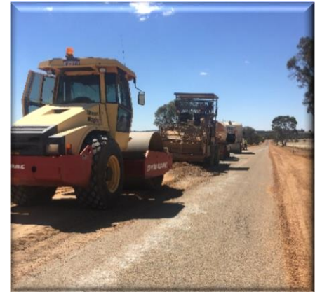
Cement Stabilising Shoulders
