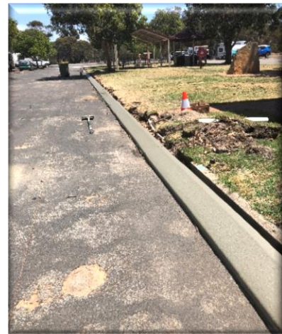
Caravan Park New Kerbing
