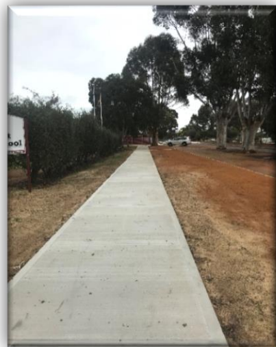
New footpath to the School
