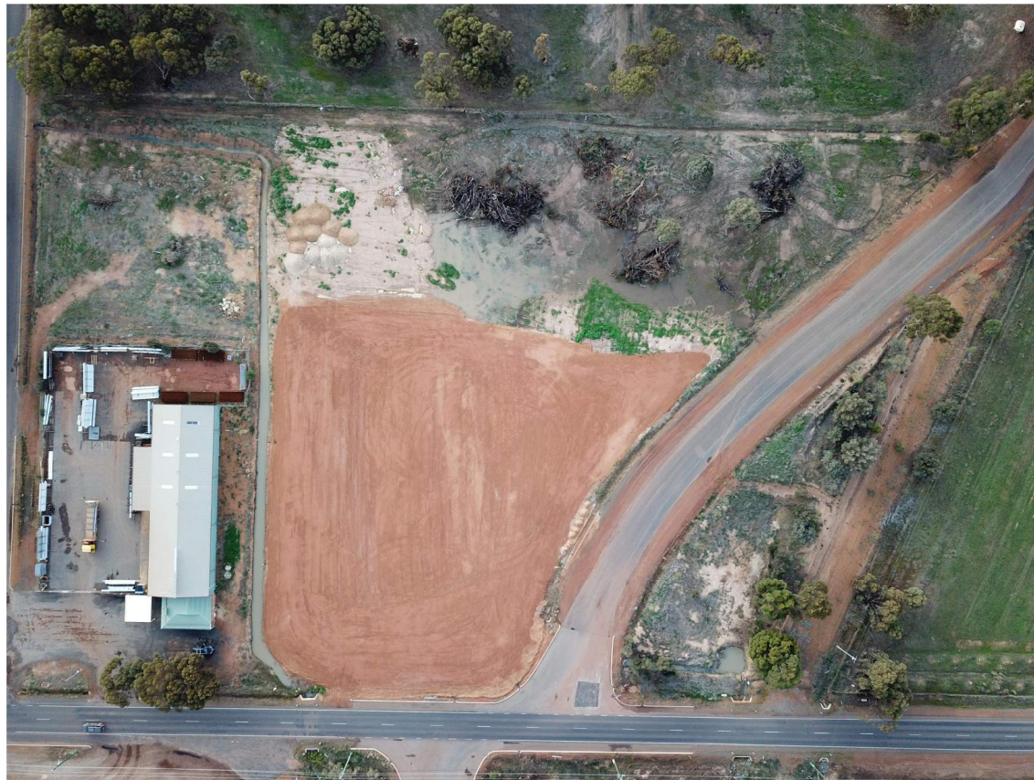
Drone Photo of the Site taken 22/06/22
