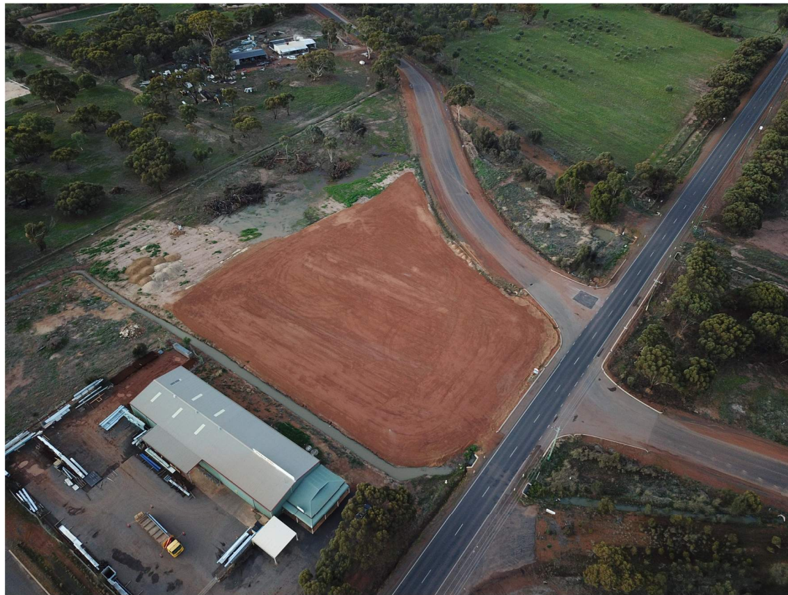
Drone Photo of the Site taken 22/06/22
