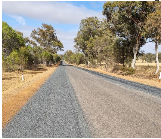
Dongolocking Road shoulder widening
