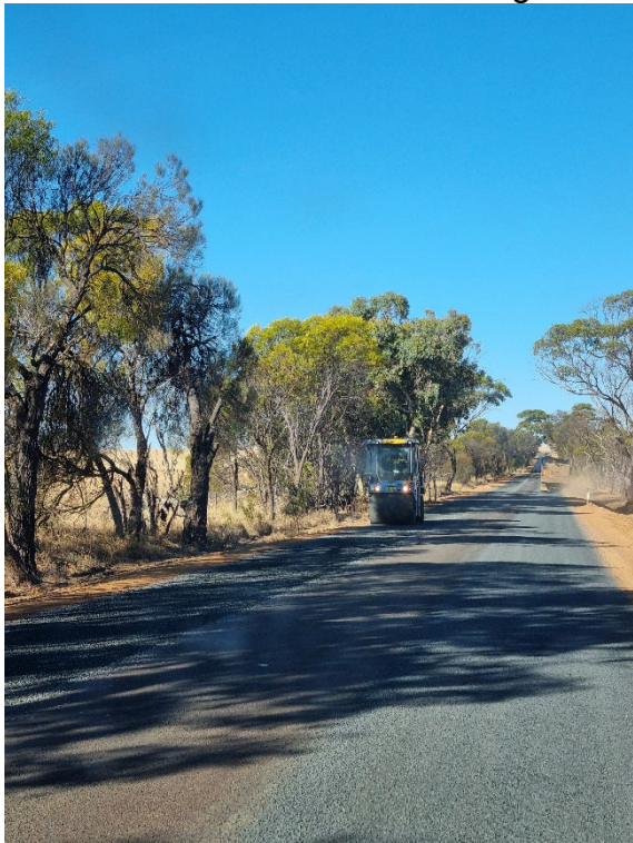
Beaufort Road shoulder widening
