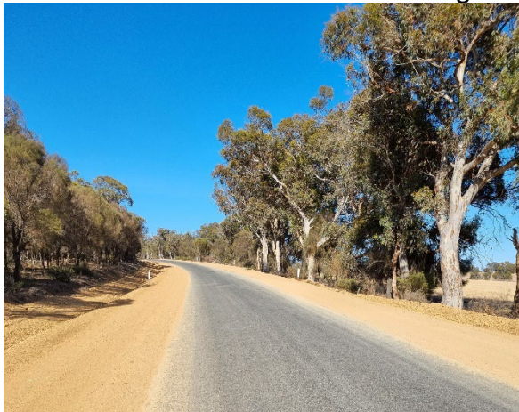
Dongolocking Road shoulder widening
