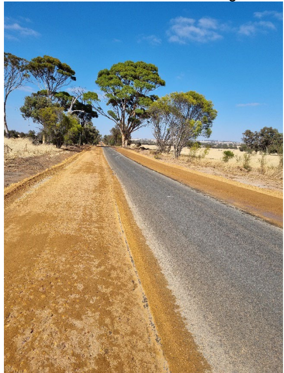
Bullock Hills Road shoulder widening
