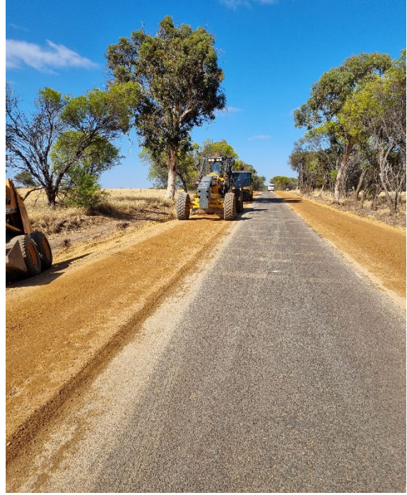
Bullock Hills Road shoulder widening
