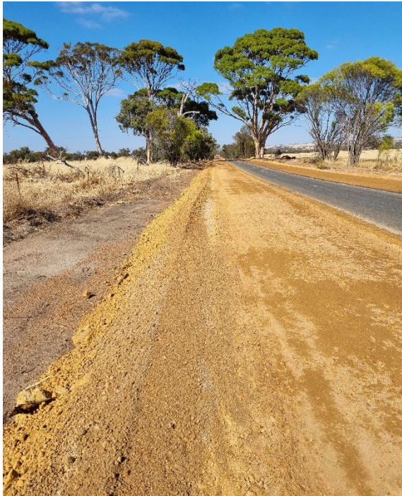
Bullock Hills Road shoulder widening
