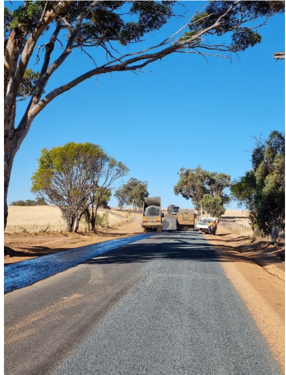
Beaufort Road shoulder widening
