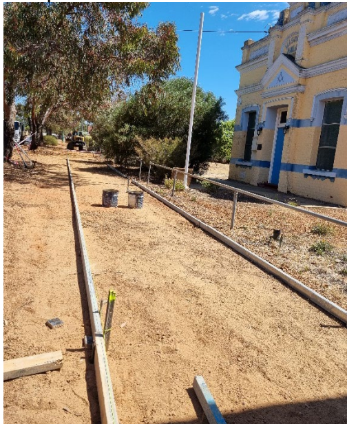
Footpath Tarbet Street
