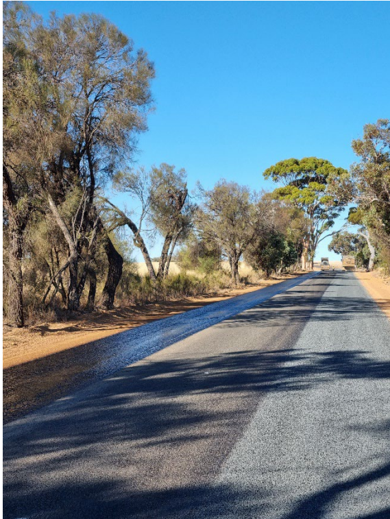
Beaufort Road shoulder widening
