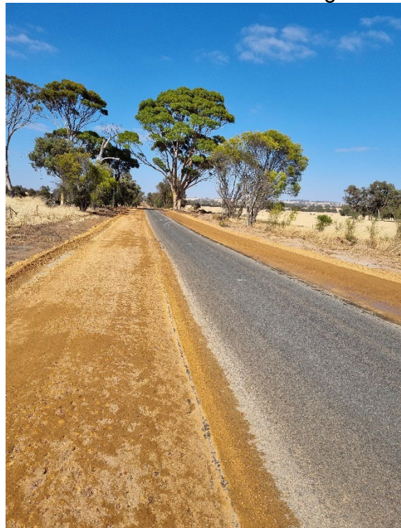
Bullock Hills Road shoulder widening
