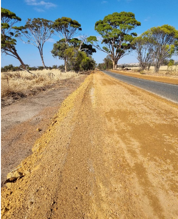
Bullock Hills Road shoulder widening
