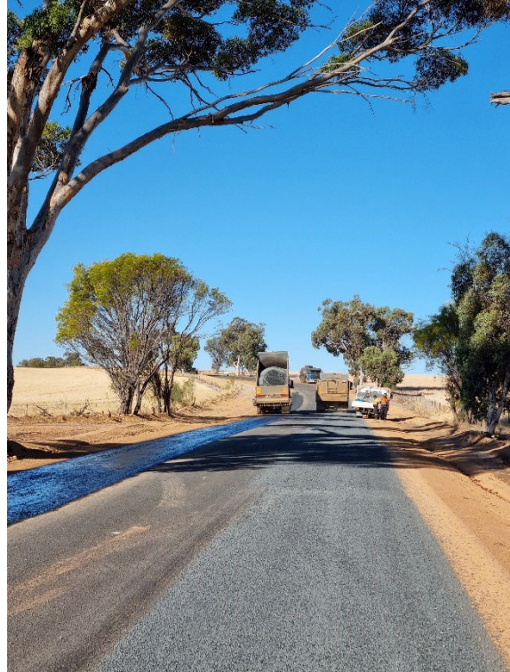
Beaufort Road shoulder widening
