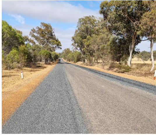
Dongolocking Road shoulder widening
