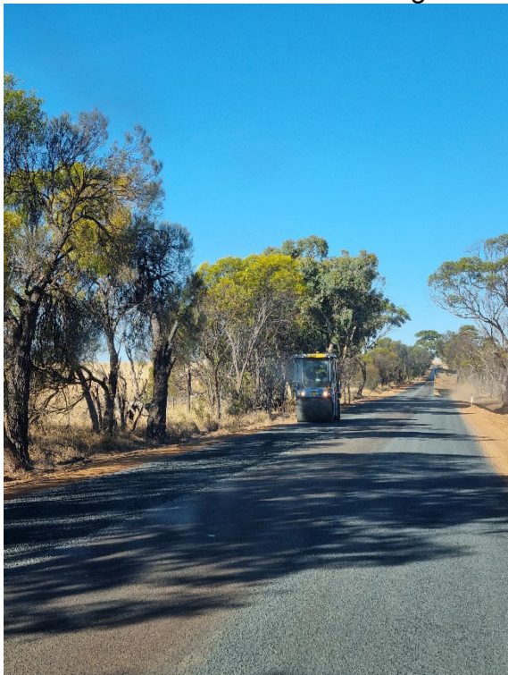
Beaufort Road shoulder widening
