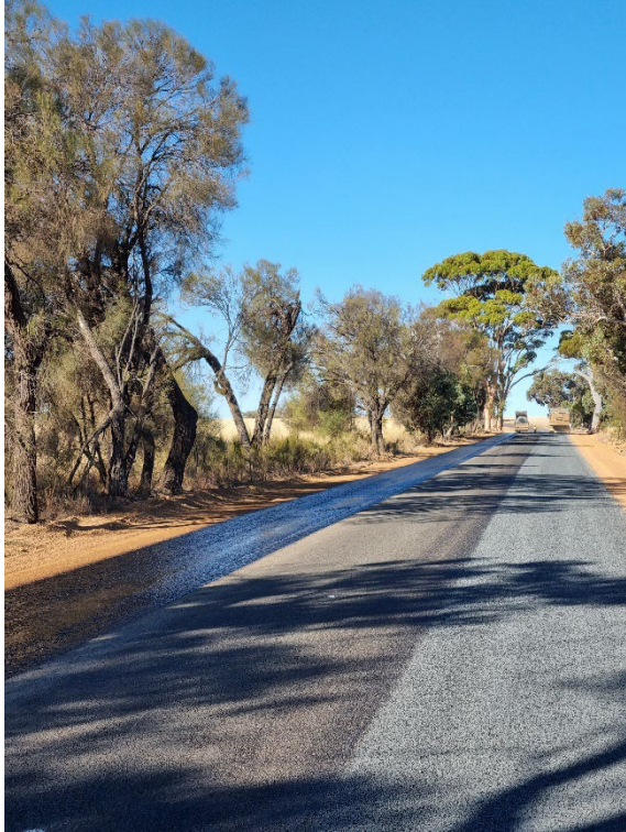
Beaufort Road shoulder widening
