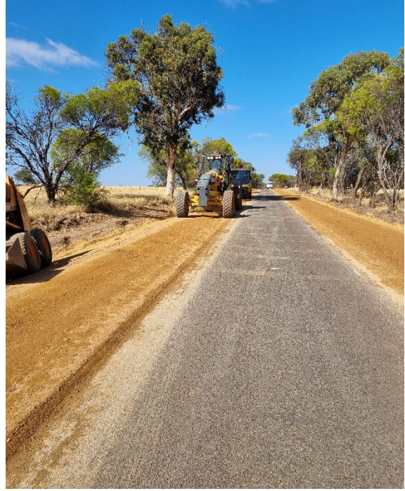
Bullock Hills Road shoulder widening
