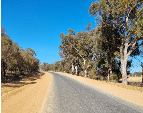
Dongolocking Road shoulder widening
