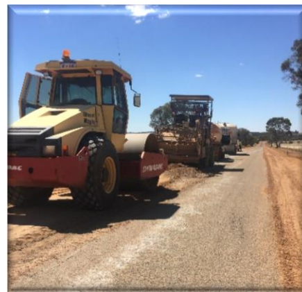
Cement Stabilising Shoulders
