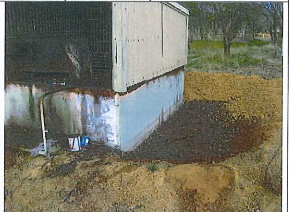
Photo 4 – Recycled waste oil facility
