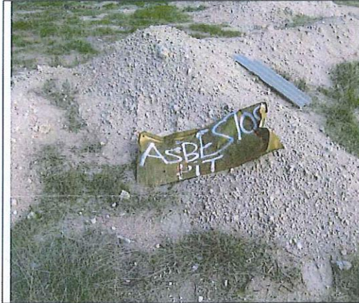
Photo 13 – Asbestos (possibly asbestos) pit sign
