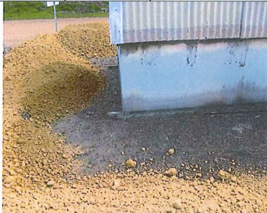
Photo 3 – Recycled waste oil facility
