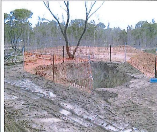
Photo 15 – Current asbestos disposal pit
