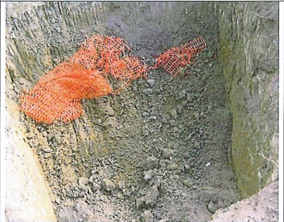
Photo 16- Current asbestos disposal pit
