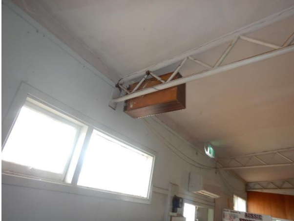
Truss connection to timber walls
