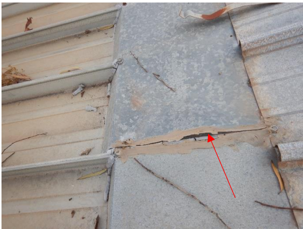
Lap failure
