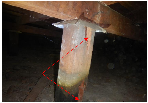
Damage timber stump
