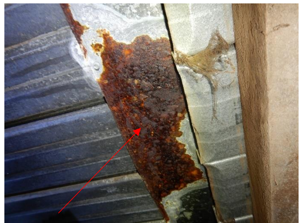
The interface flashing between original and addition is failing
