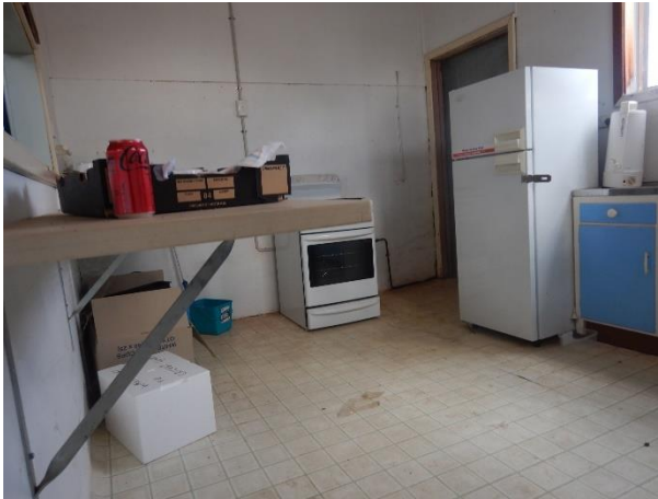
Vinal floor covering cement sheeting to walls and ceilings
