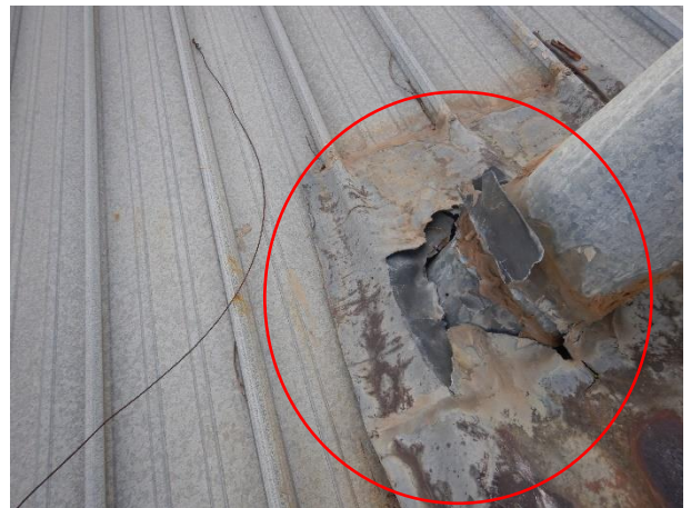
Flue failure/lead flashing
