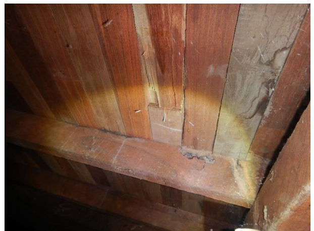
Termite damage to flooring
