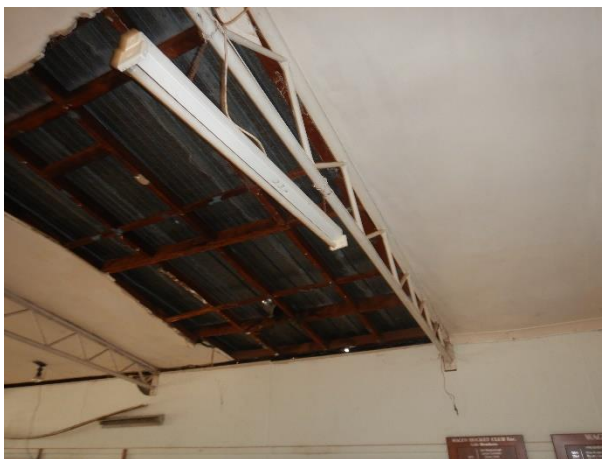
Failed ceiling at flue
