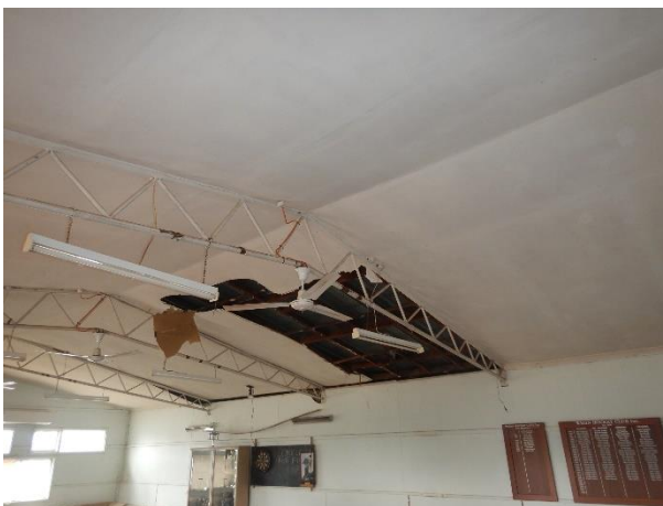
Typical steel trusses
