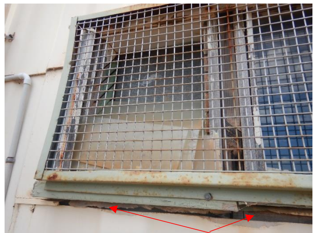
broken louvers and water entry point
