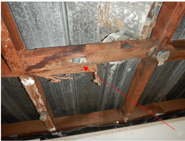
Termite damage to the purlin
