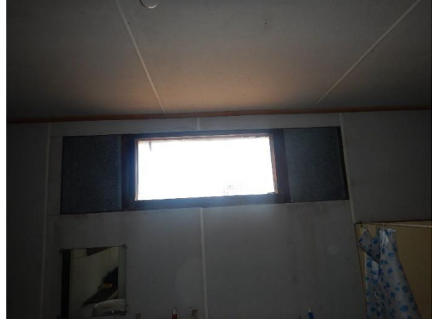
Typical ceiling/wall cement sheeting
