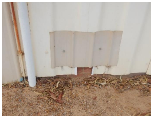
Typical repairs to existing cladding
