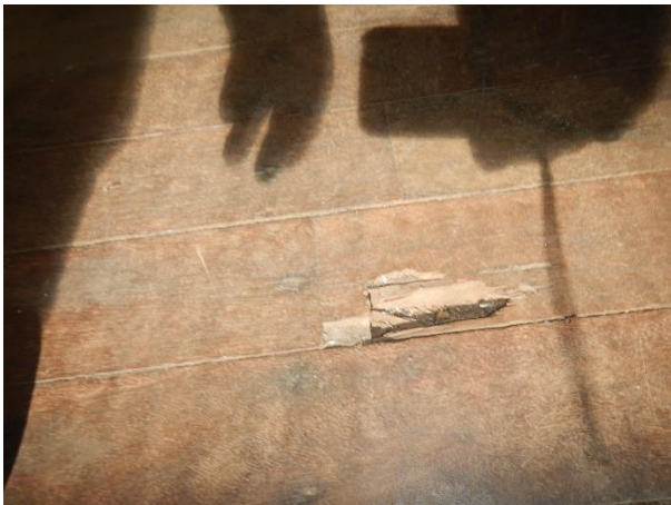
Termite damage to flooring
