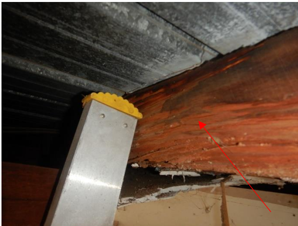
Termite damage around flue
