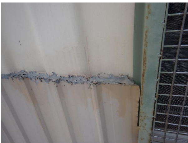
Typical repairs to existing cladding
