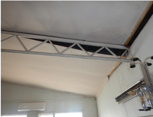
Failed ceiling due to glue failure (Typical)
