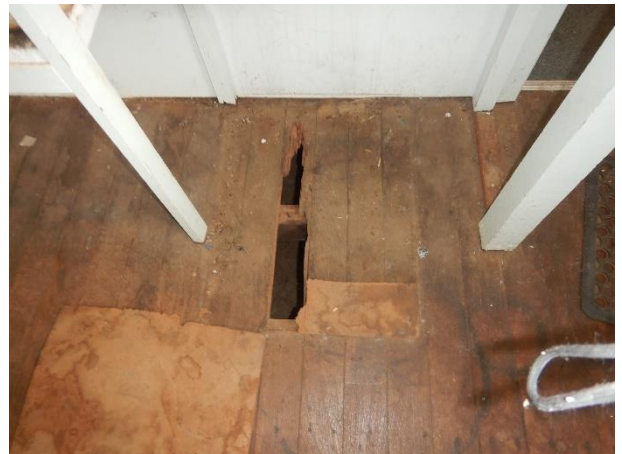
Termite damage to flooring
