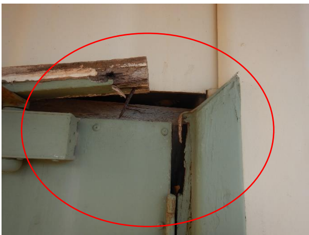
Door frame head failure
