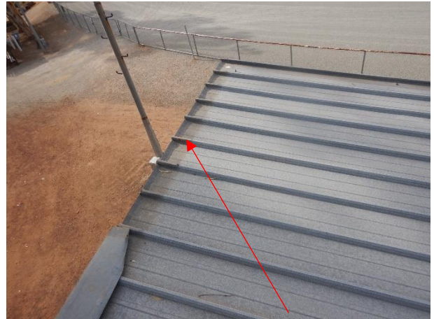
Barge flashing missing
