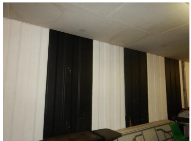
The original Asbestos wall cladding
