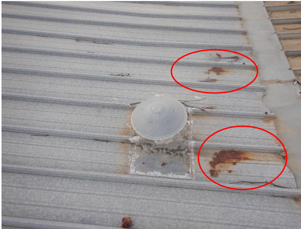
Corrosion to these sheet ends
