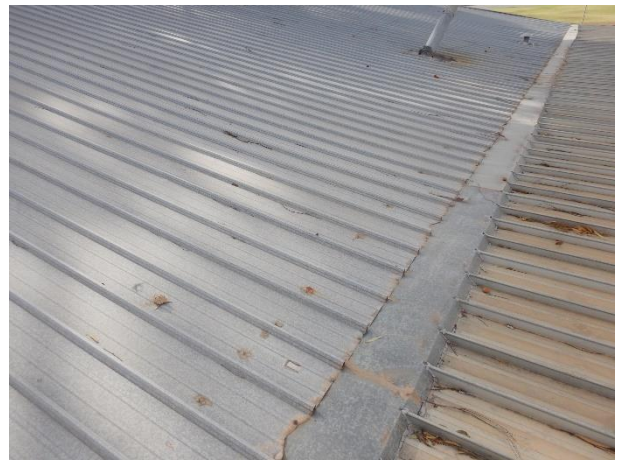
Interface between the original and addition
