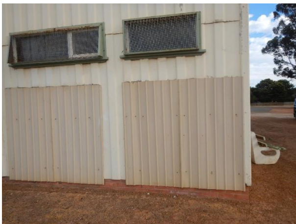
Typical repairs to existing cladding
