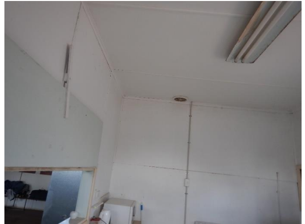
Vinal floor covering cement sheeting to walls and ceilings
