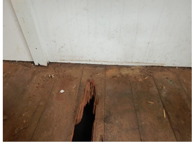
Termite damage to flooring
