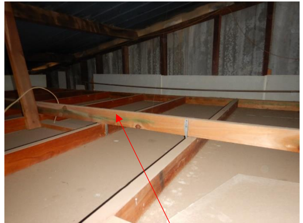
Ceiling frame, (Hanger should be minimum 190x35)
