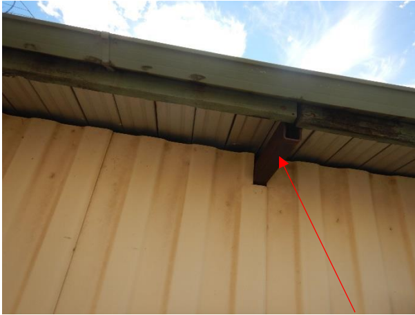
Eastern extension RHS roof supports and timber purlins
