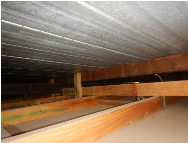
Ceiling frame appears fit for purpose.
