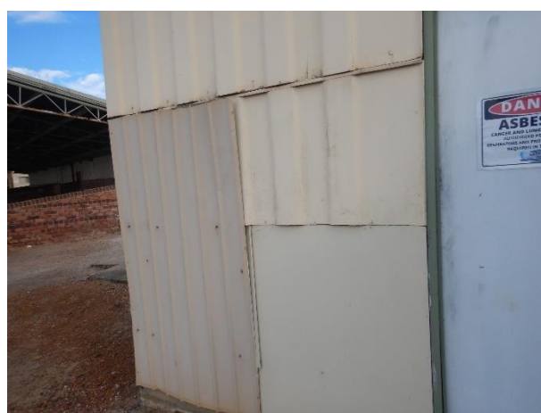
Typical repairs to existing cladding
