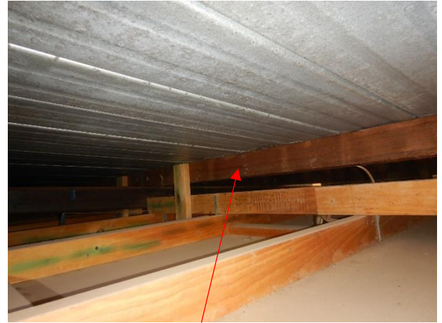
Eastern extension RHS roof supports and timber purlins
