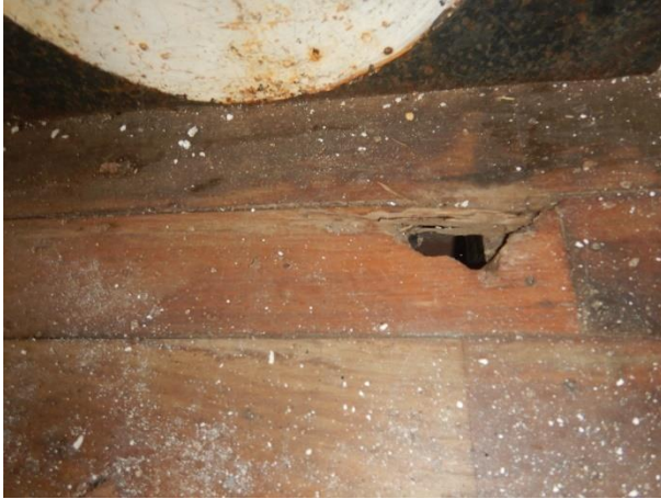
Termite damage to flooring
