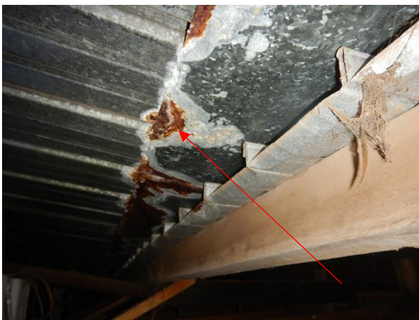
The interface flashing between original and addition is failing
