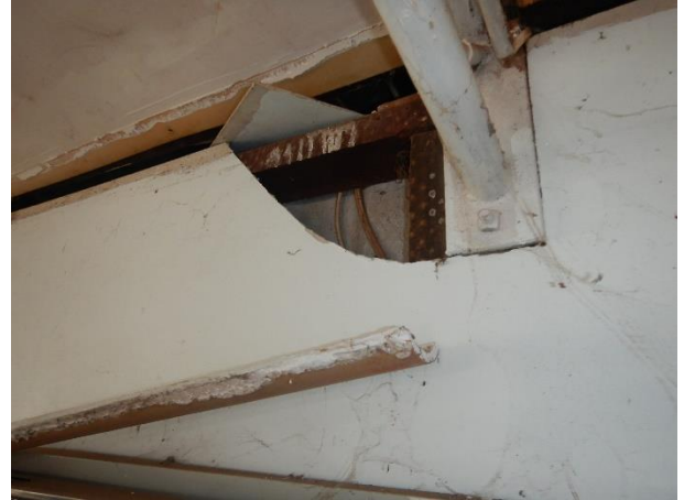
Truss connection to timber walls
