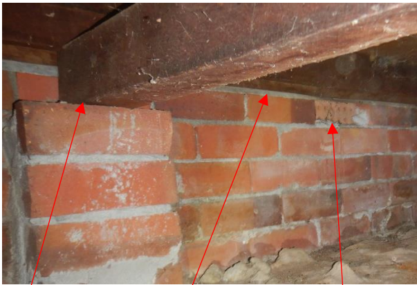
No ant cap here Ant cap here Brick vent
