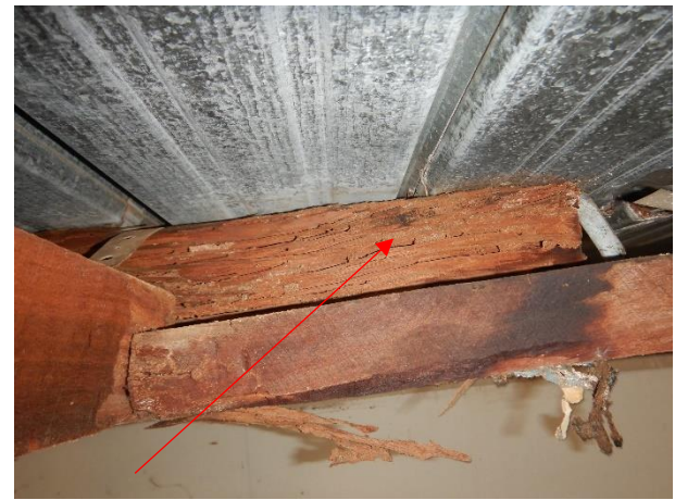
Termite damage to the purlin
