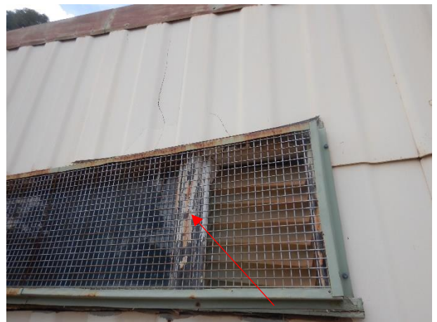
Timber frame is no longer viable
