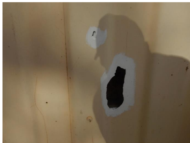
Typical repairs to existing cladding
