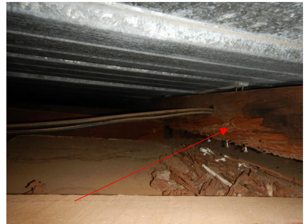
Termite damage around flue
