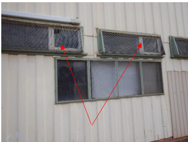
These timber windows are no longer serviceable
