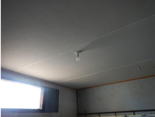
Typical ceiling/wall cement sheeting
