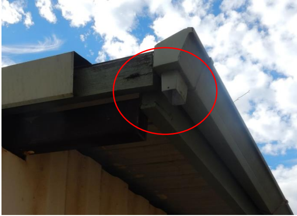
Stormwater discharging straight onto the ground
