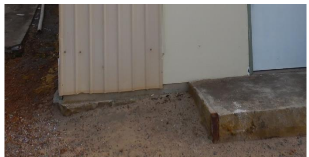
External slab edge to eastern addition
