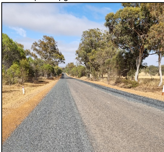
Stabilising works to Dongolocking Road
