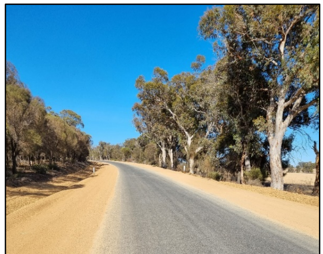
Shoulders widened Dongolocking Road
