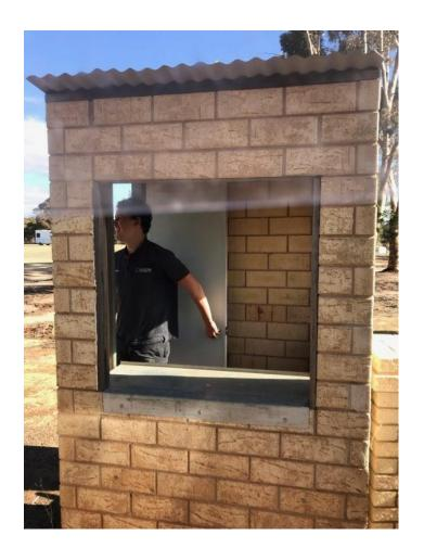
It was agreed that a permanent ticket box structure was required on the southern entrance of the main Spoertsground entrance. The structure to be built in brick with a colorbond roof. The building to provide a place to sell tickets from both the pedestrian side gate and the vehicle entrance. The structure will also provide shelter over the pedestrian acess.
