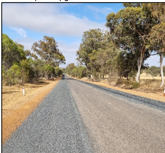
Stabilising works to Dongolocking Road
