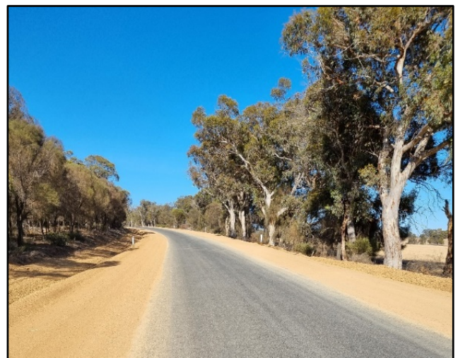
Shoulders widened Dongolocking Road
