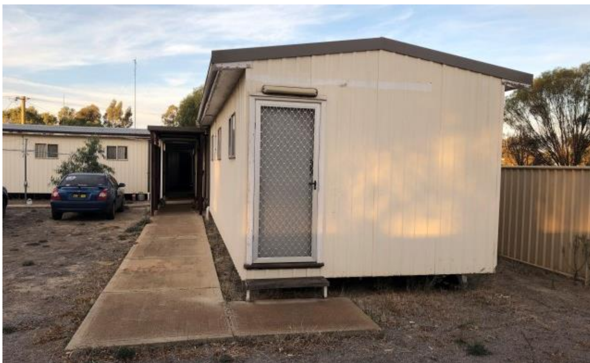
Photograph 1 – Portion of the existing development
