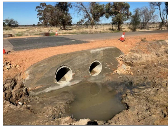
Culvert replacement – Beaufort Road
