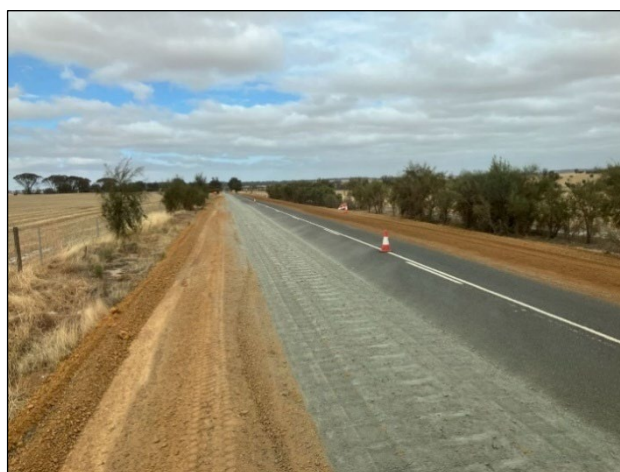
Stabilising works on Bullock Hills and Ballagin Roads
